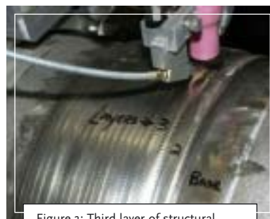
Figure 3: Third layer of structural weld overlay
