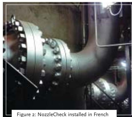
Figure 2: NozzleCheck installed in French nuclear power plant
