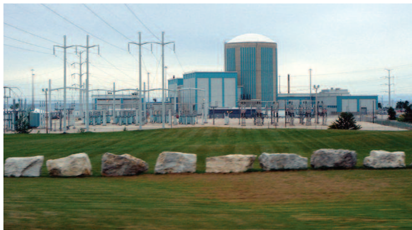
Kewaunee Nuclear Power Station
