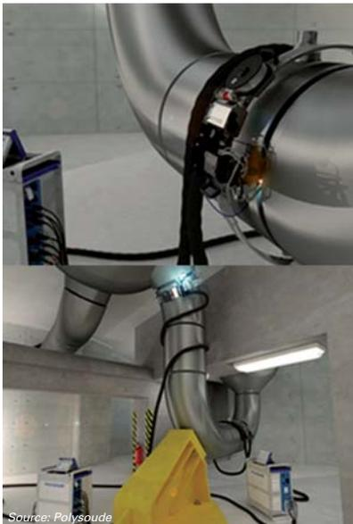
Fig. 4. Primary coolant circuit orbital NG welding.
