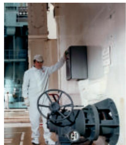
*Typical outside containment installation of Rotork Nuclear actuator.*
