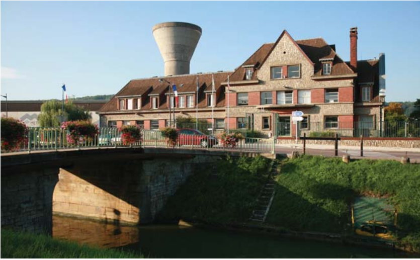
The company has a long history in Europe dating back over 120 years; this is the administration building at the production site in Montbard, France.
