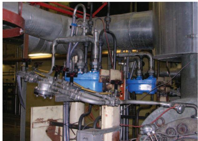
The original seal cooling system (left) and the new optimized seal cooling system
