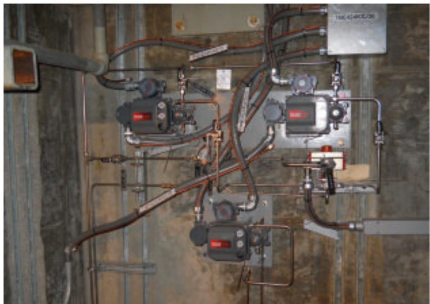
*Figure 2: Remote mount DVC electronic units shown on panels.*
