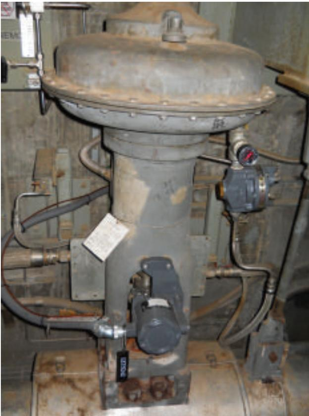
*Figure 3: New non-contact feedback sensors mounted on feedwater bypass valves.*
