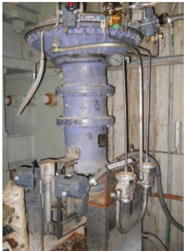
*Figure 4: New feedback sensors mounted on main feedwater regulation valves-dual redundant system.*
