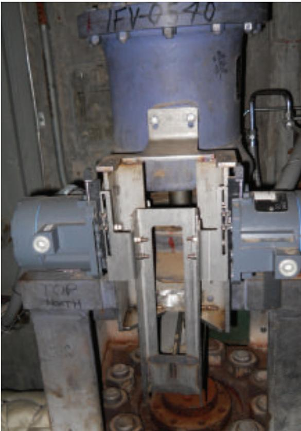
Figure 5: New feedback sensors on main FW reg valves-close up.
