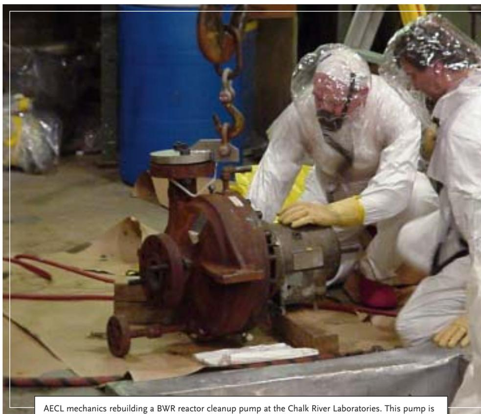
AECL mechanics rebuilding a BWR reactor cleanup pump at the Chalk River Laboratories. This pump is highly radioactive and must be handled with care. Without reliable operation of this pump, the reactor cooling system chemistry would slowly deviate from specification forcing a plant shutdown.
